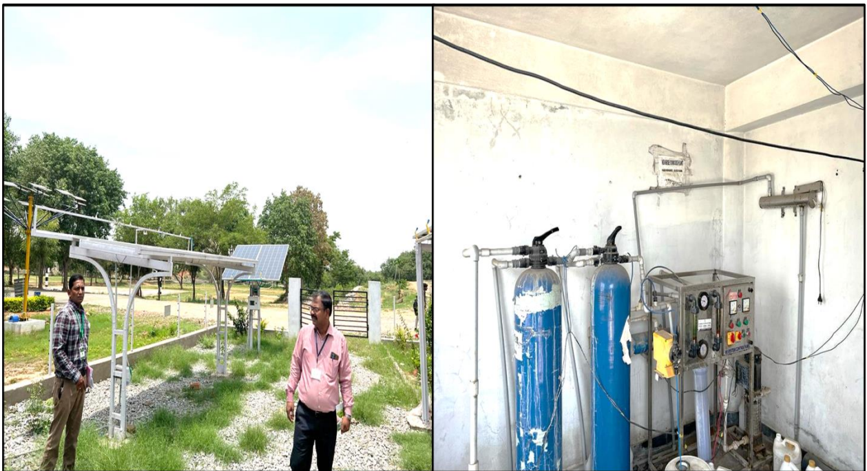
RO Water and Solar Panels observed Bharat Institute of Engineering & Technology, Hyderabad, Telangana
